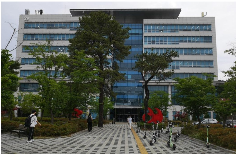
DaVinci hall – building where Industrial Design programs are held.
